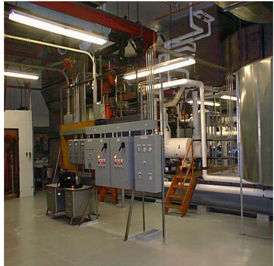
Cooling Tower - After
