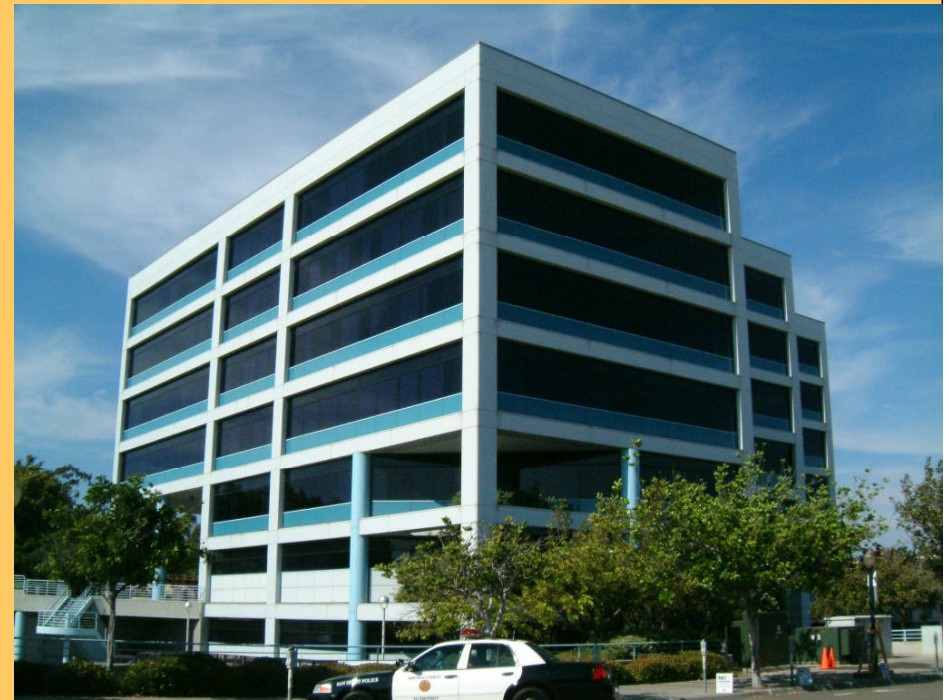
San Diego Police Dept HQ Bldg ESCO: Onsite Energy
