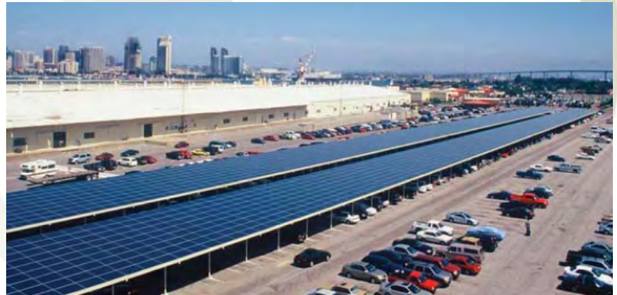
Chevron/PowerLight 924kW Parking Structure US Naval Base, Coronado CA
