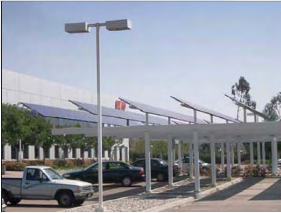
Elevated one-axis tracking PV
